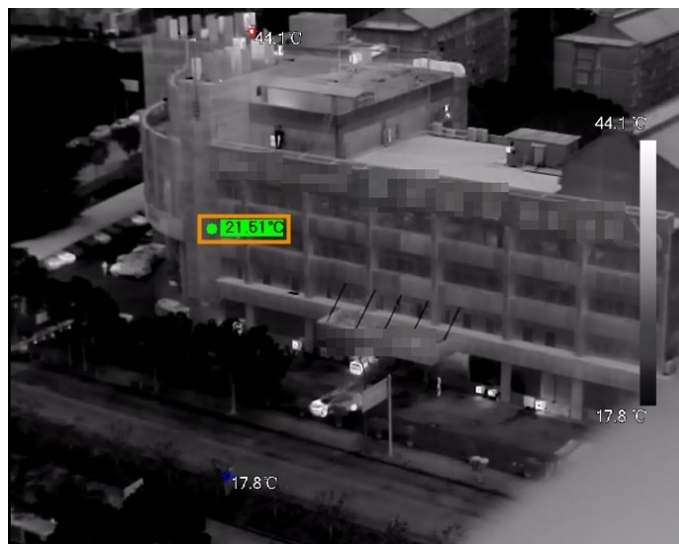
Figure 4-6 Real-time spot temperature measurement
